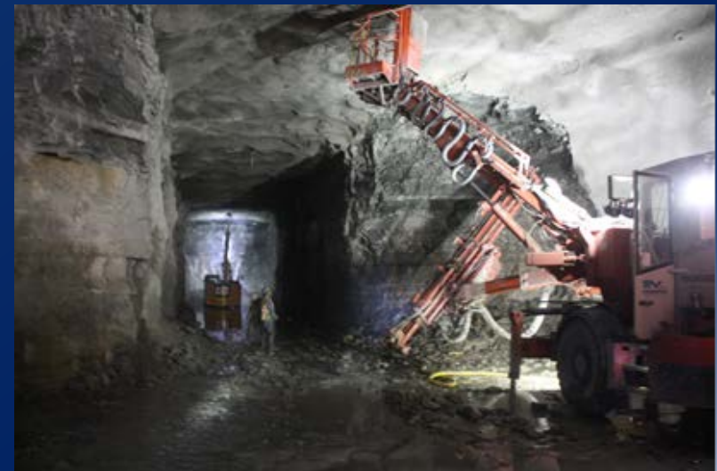
f) Sequential excavation method in relatively weak rock (center, 2 side [L & R] headings & bench)
