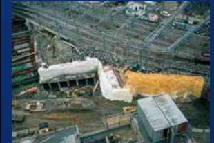
c) Jacked Tunnel
